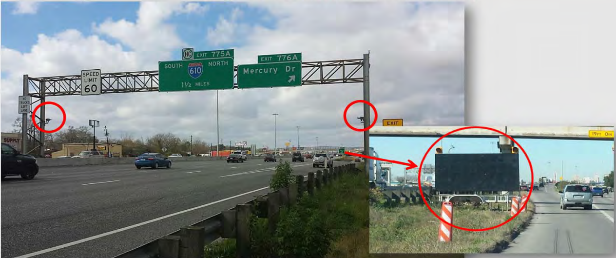
Detectors installed on OSB in Advance of Low Clearance Bridge
